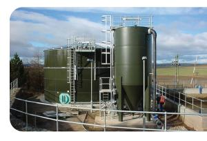
Evoqua's DAVCO Continuous Backwash Filter is an ideal technology for tertiary nutrient removal
