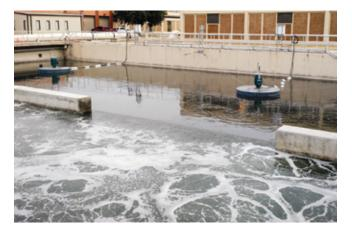
Aqua-Lator<sup>®</sup> Direct Drive Mixers are an ideal solution for anaerobic and anoxic tank mixing in wastewater treatment applications.
