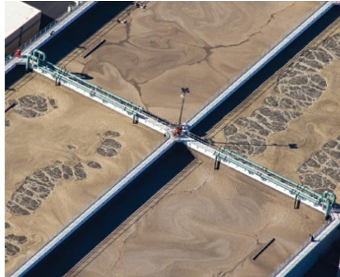
The OMNIFLO SBR MAX control system automatically adjusts to the flow coming in, giving the operators the best of both worlds: true-batch handling at design flow and optimal hydraulic handling at storm flows.
