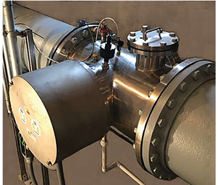
Evoqua's ETS UV closed vessel medium pressure SW-1250-20 UV reactor
