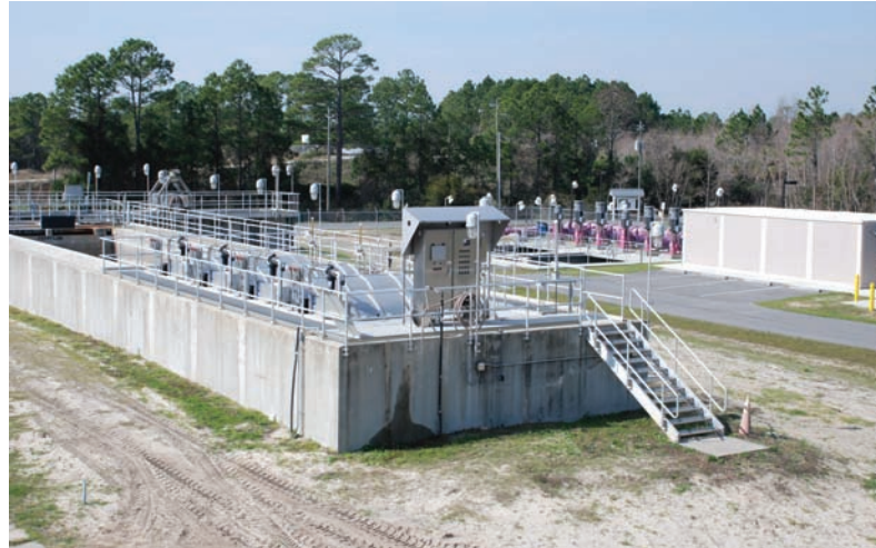
The complete disc filter retrofit is shown on-site in the foreground, with the reuse pump system that transfers the treated water to Conservation Park in the background.
